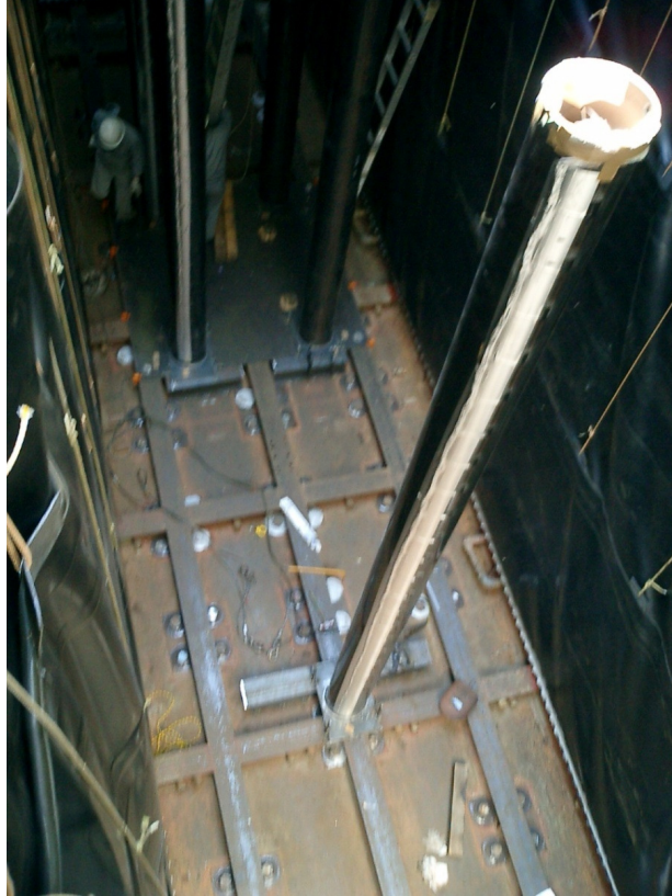
Figure 2.3. NIED, Tsukuba, Japan, 5m high Single Test Pile (Elgamal 2008)
