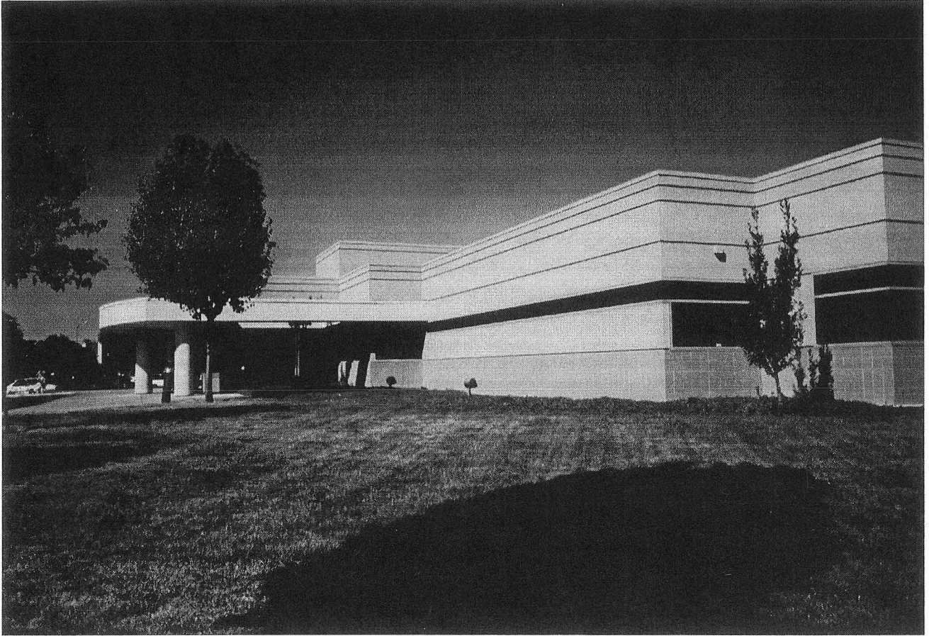
Figure 1(a): Ground-level view of the Davis building
