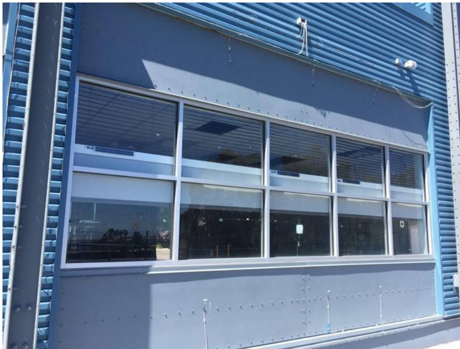
Figure 5. External view of FLEXLAB testbed with INTER shading system installed
