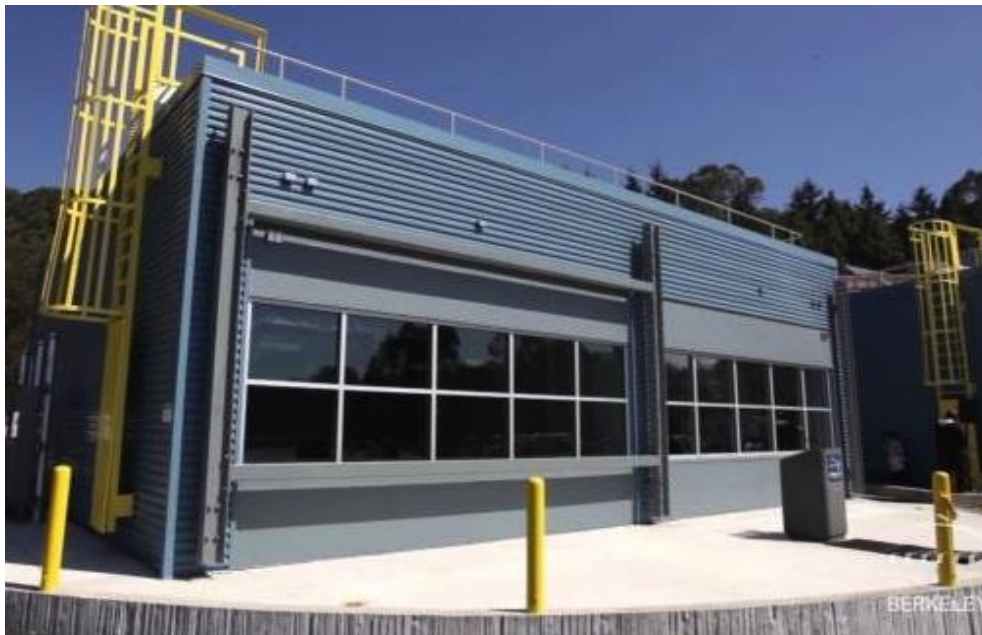
Figure 3. External view of a FLEXLAB testbed
