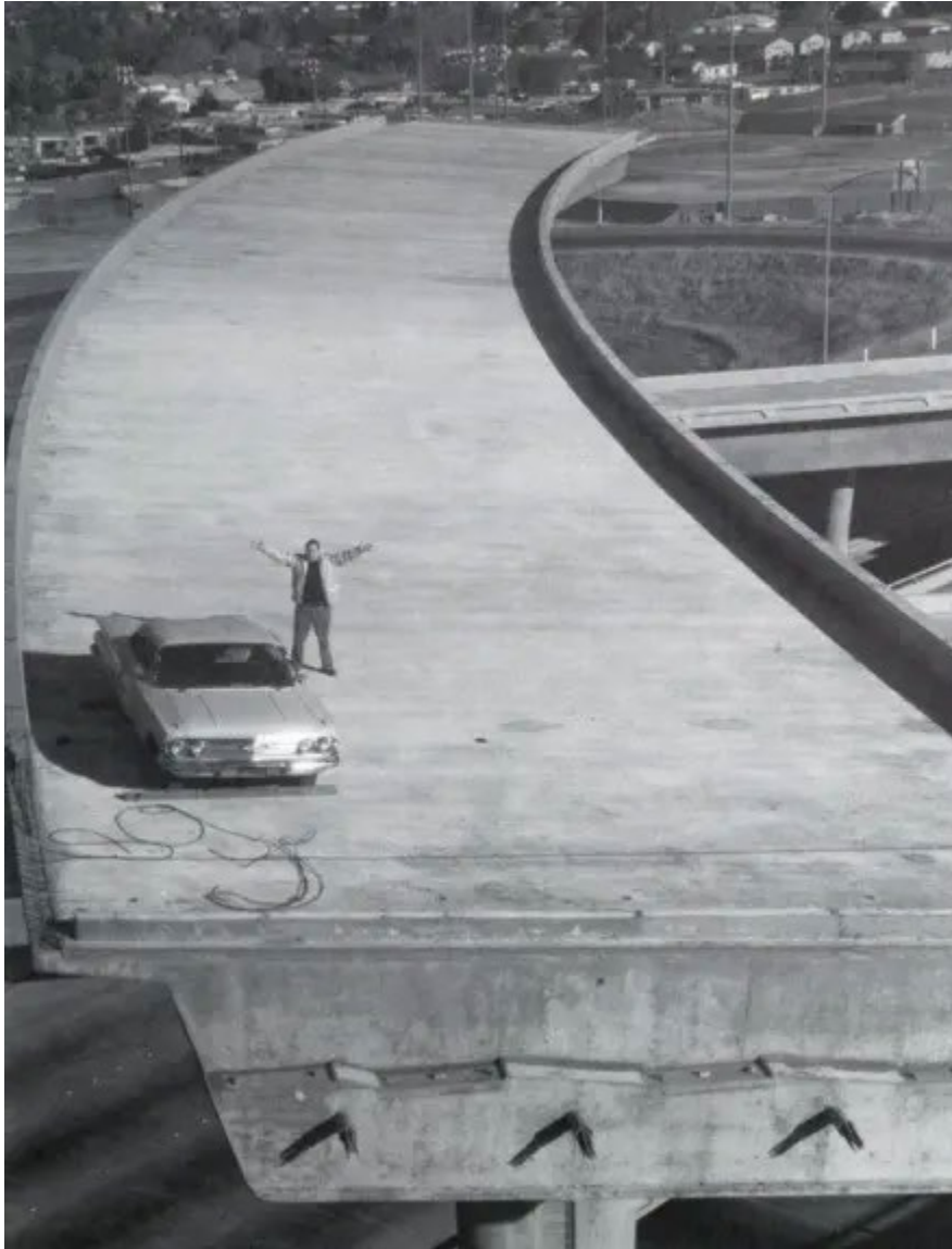
Figure 8-13. Joe Colla atop the Unfinished US-101/I-280/I-680 Interchange
