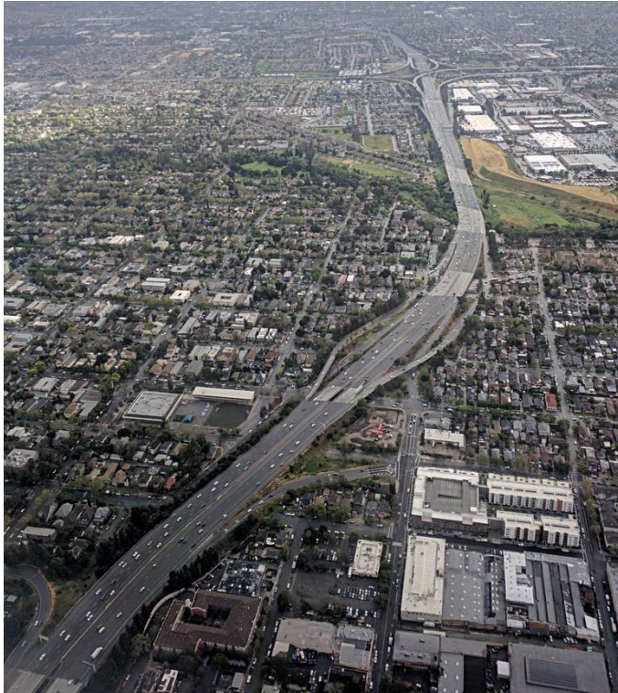
Figure 8-9. Sinclair Freeway/I-280 at US-101
