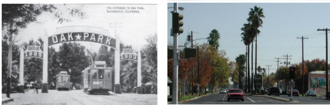
Figure 7-14. Corner of Broadway and Alhambra Boulevard, the Entrance to Oak Park, 1910 and c. 2005
