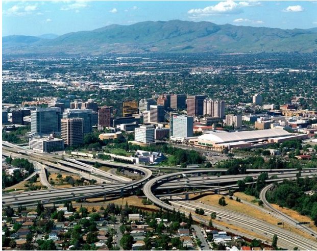
Figure 8-3. Downtown San José and Interchange of I-280 and SR-87
