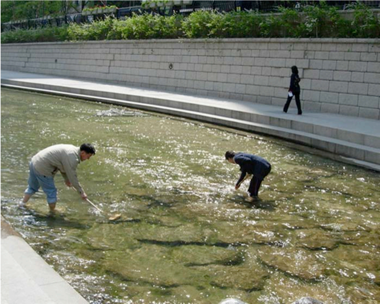
Figure 27. Workers scrub the algae off the rocks and bottom of the Cheonggyecheon (François Rejeté).
