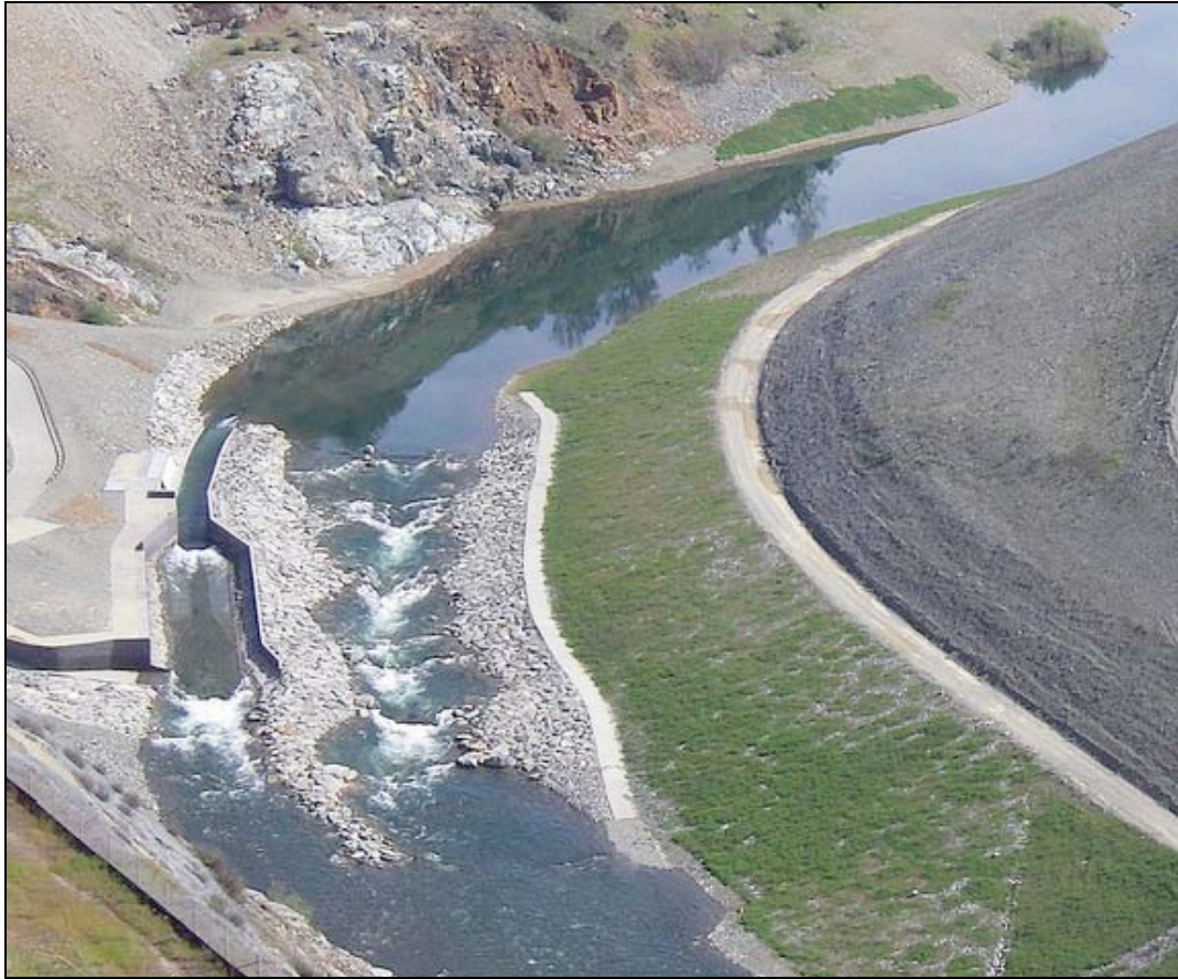
Figure 39. A multifunctional fish passage, water diversion, and whitewater design on the American River in Auburn, California. The whitewater channel or hydraulic chute channel is to the right in the image. Photo compliments of McLaughlin Water Engineers.
