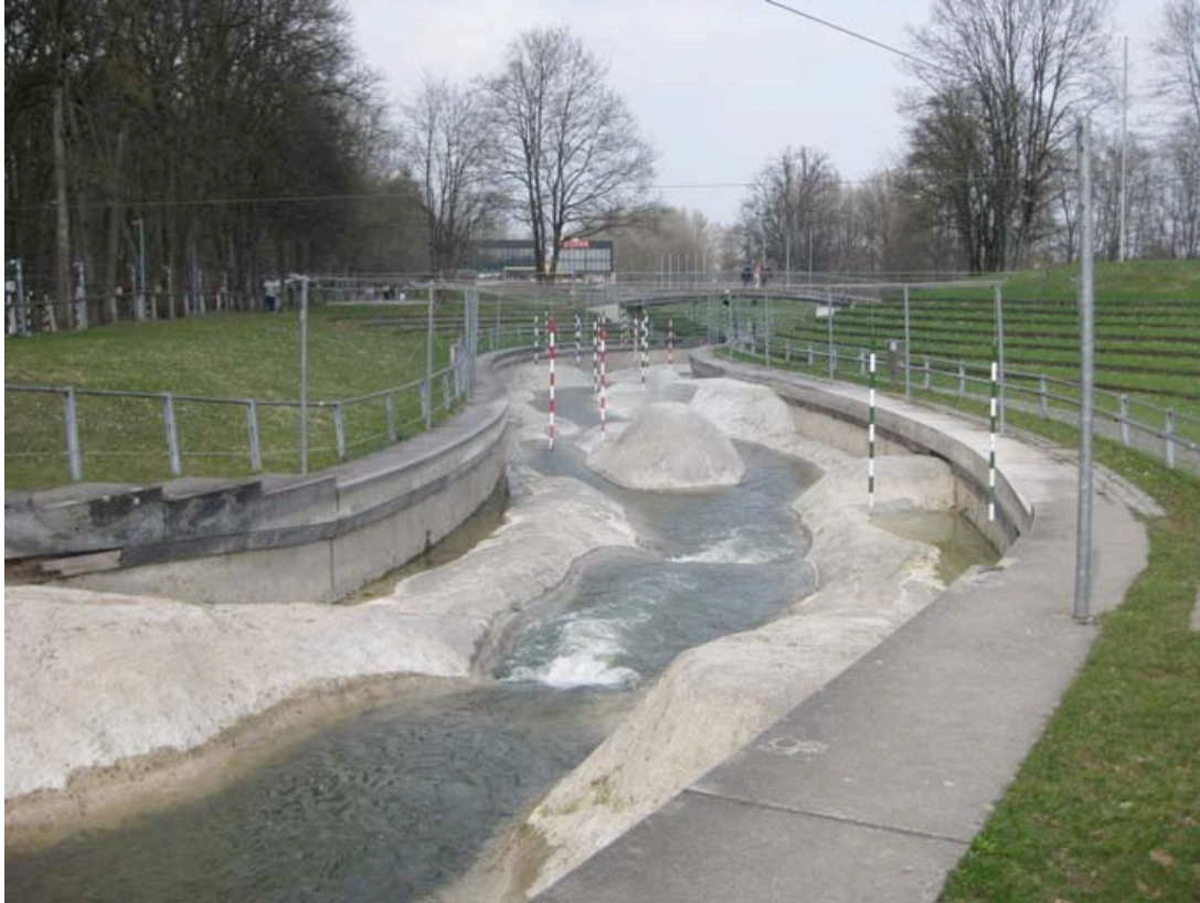
Figure 32. The 1972 Augsburg Olympic whitewater slalom course with low water flow showing the shape of the channel bottom. Photo by Thorsten Hartmann.
