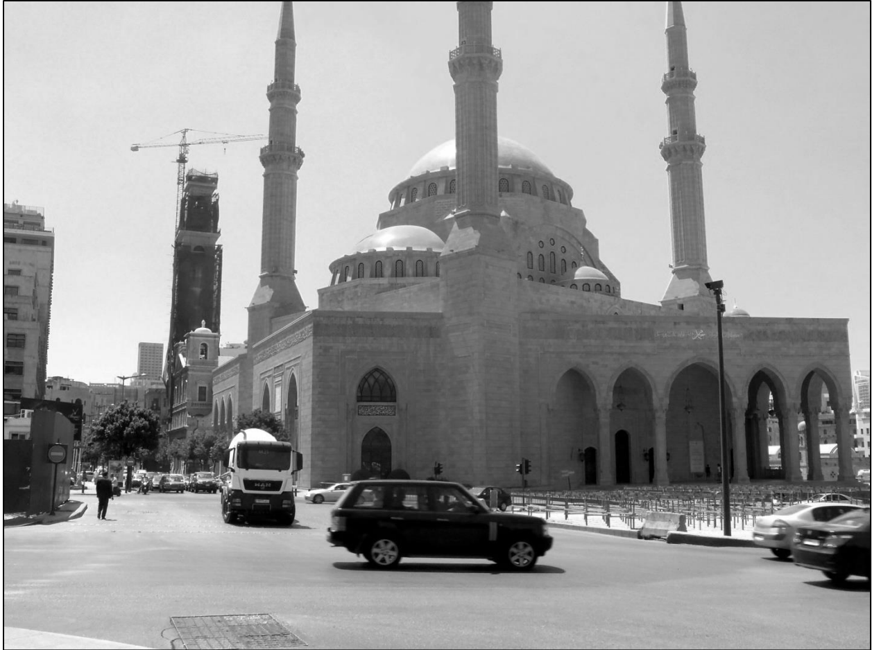
4. Southwest corner of Martyrs Square: Hariri Mosque (foreground) and St. George's Maronite Cathedral with bell-tower (back left).
