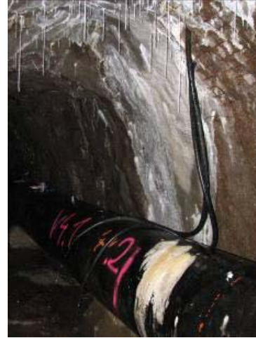
Figure 3-6. Bohemian granitic massif in Czech Republic and Water Inflow Evidence in the Bedrichov Tunnel (from Hokr and Slovak, 2011)
