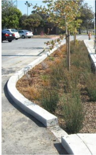
Figure 4-30: Bioretention Curb Bulb-out
