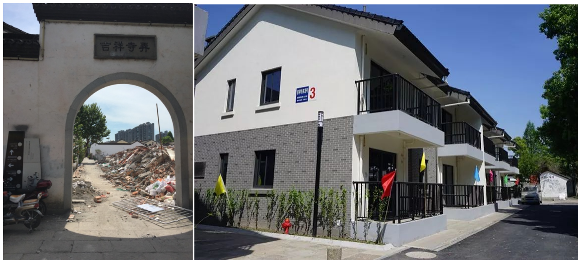
Figure 4- 9: (Left) Jixian Lane undergoing demolition in 2017. Photography by the author. (Right) Image of Jixian Lane after reconstruction. From J. Wu (2019).
