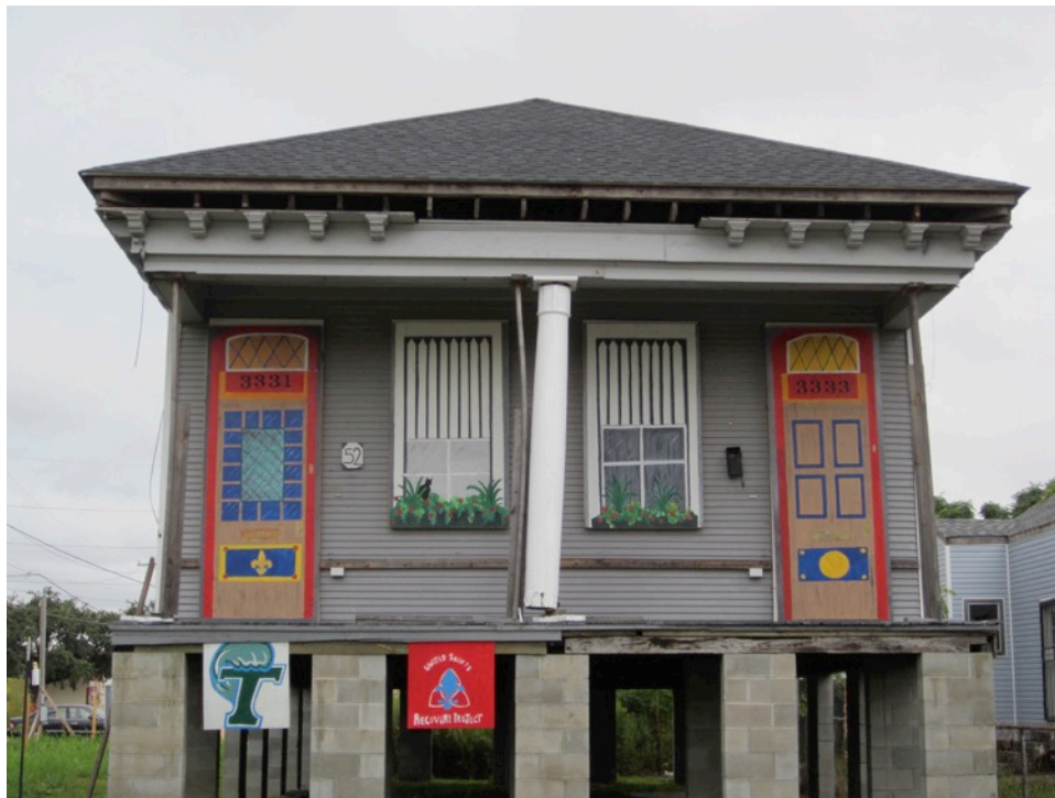
Figure 30. A vacant house painted to look like it is occupied. Photo by author. 2013.
