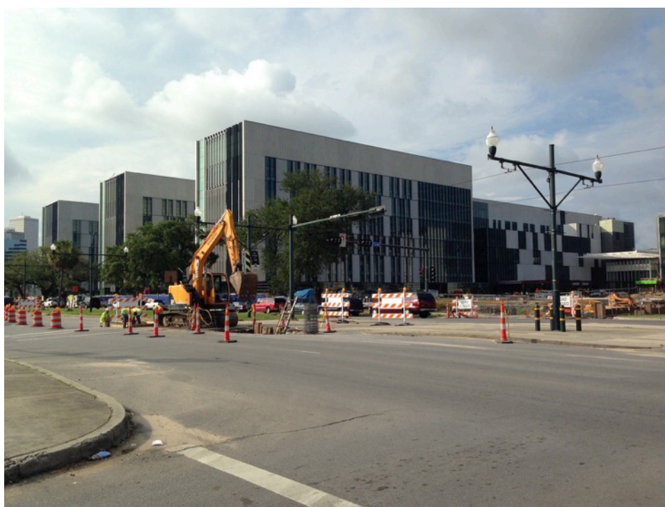
Figure 5. Hospital about a year away from completion. Photo by author. 2014.
