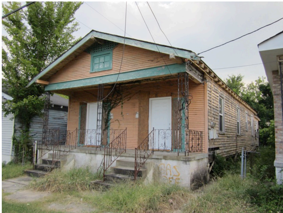
Figure 15. The house with new doors. Photo by author. 2011.
