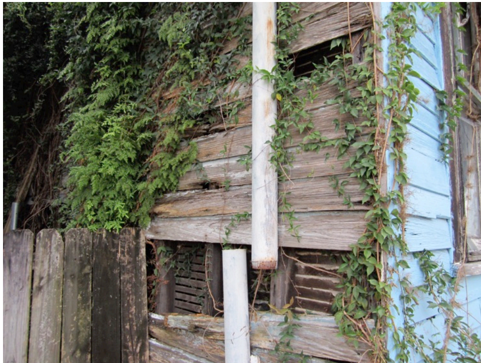
Figure 20. Vines growing through a house. Photo by author. 2013.
