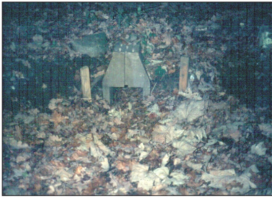
Figure 7. Main causes of malfunctioning amphibian mitigation measures I.: lack of maintenance (Henley-on-Thames, England).
