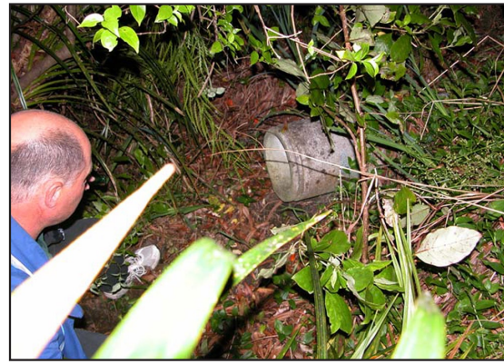
Figure 8. Main causes of malfunctioning amphibian mitigation measures II.: construction problems (tunnel entrance over the ground), besides the fence is lacking (near Auckland, New Zealand). (Photo courtesy: Dr. Phil J. Bishop)
