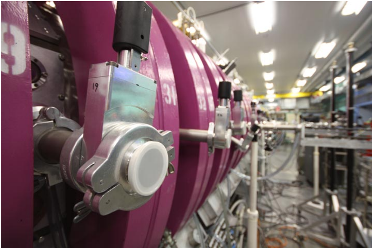
Figure 3.4: Close-up of a typical vacuum feed-through for insertion of a diagnostic probe.
