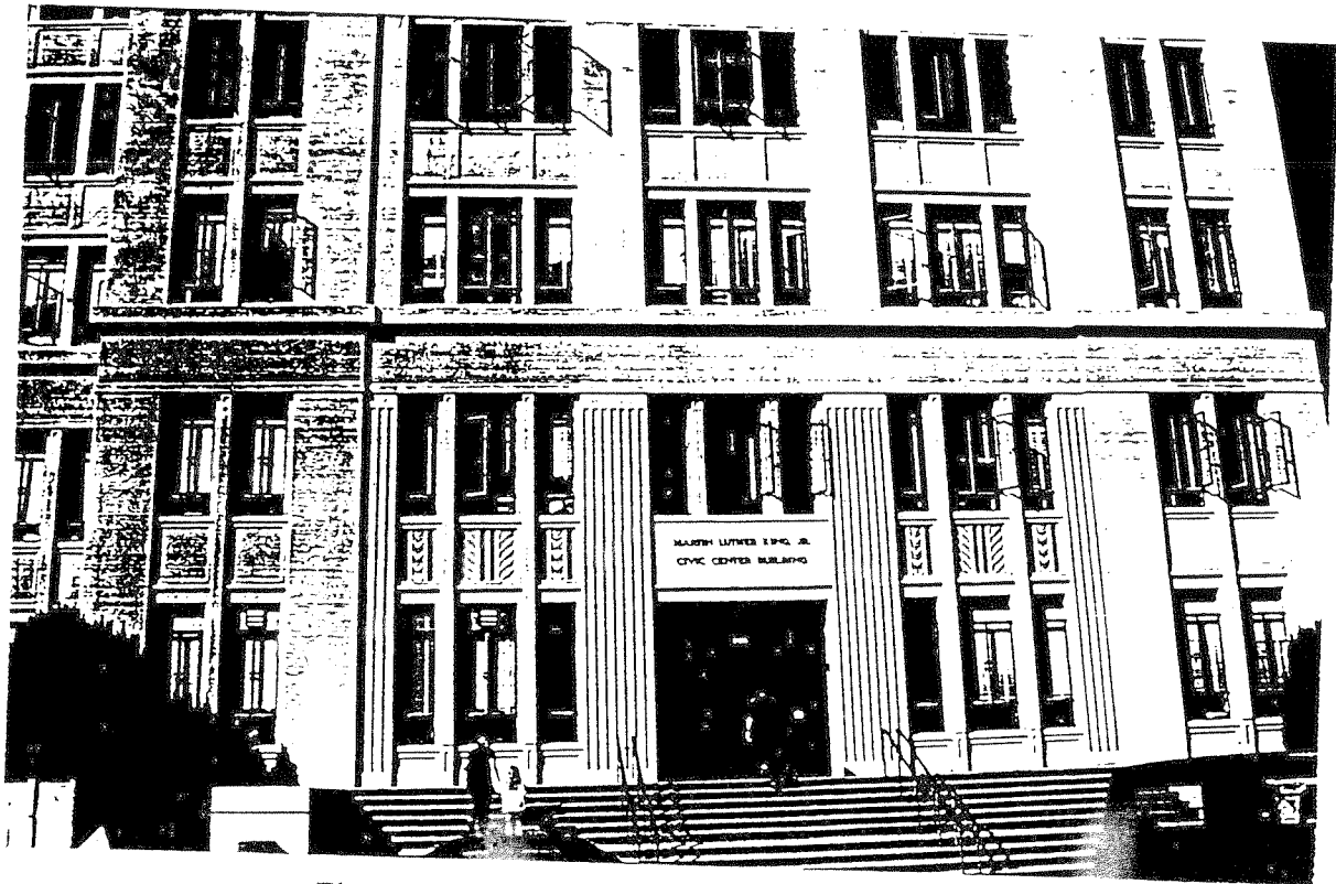
Figure 1a: Front View of Berkeley Civic Center
