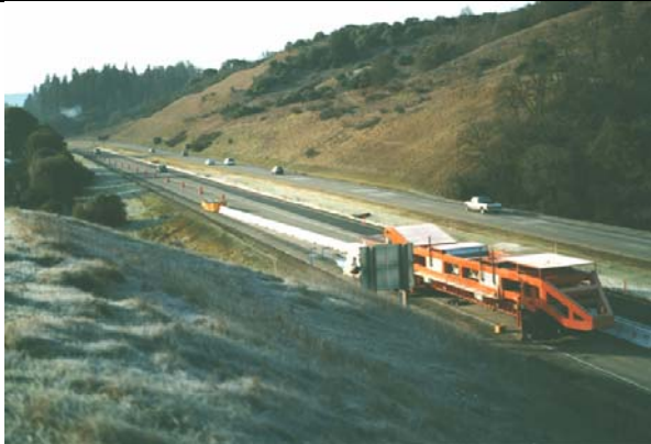
HVS2 on US-101 dowel bar retrofit sections, Ukiah, California, 2001
