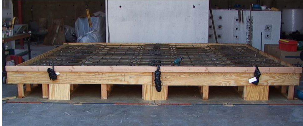
(a) Construction of specimen formwork
