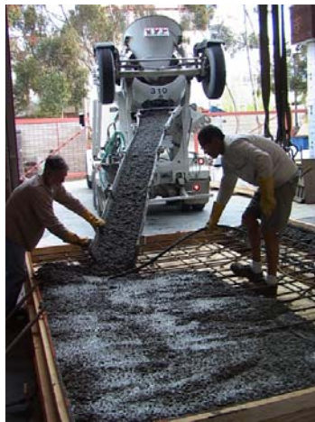
(b) Pouring of concrete and finishing of specimen surface
