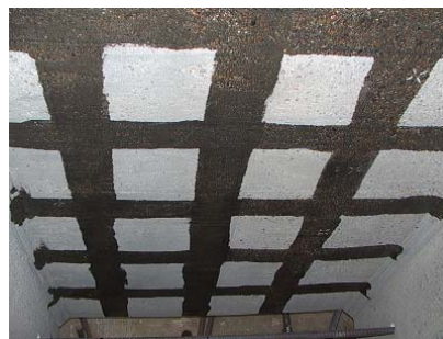
b) Primed surface for composite installation
