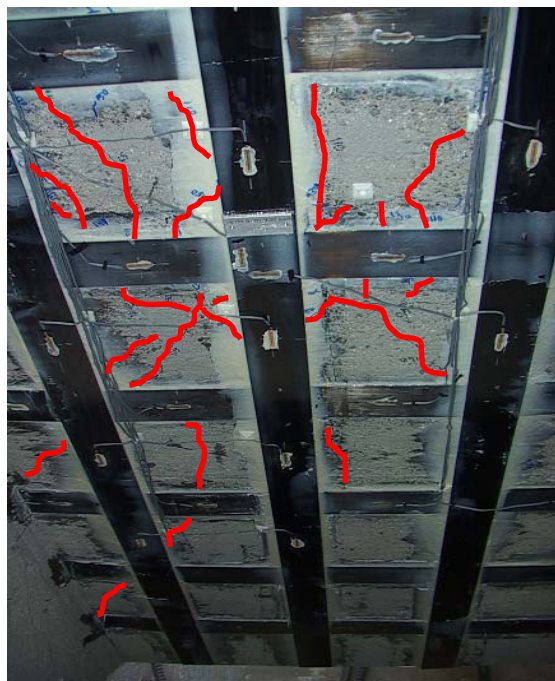
Slab 1 with pultruded strip system
