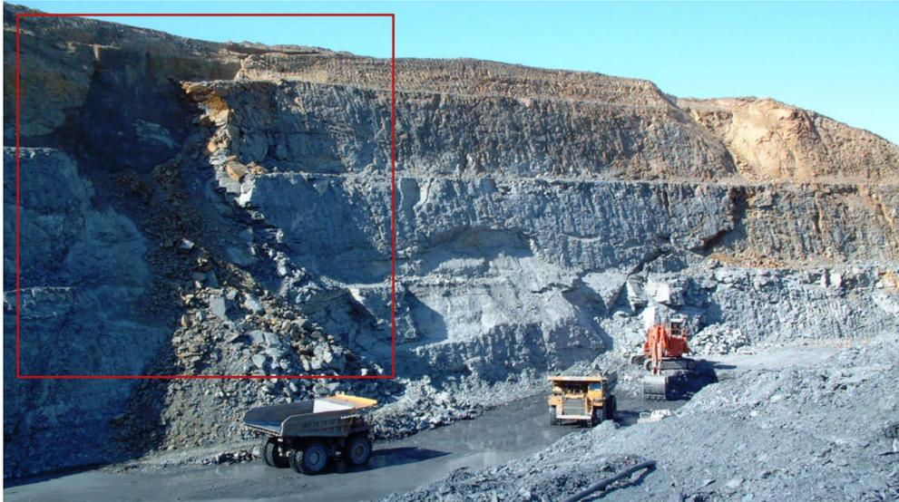
Figure 4.1: Round Hill open-pit mine failure
