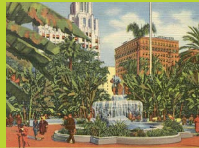
1951 Popular, lush, yet "seedy" Pershing Square in Downtown Los Angeles undergoes renovation to dissuade undesirable behaviors - including homelessness. After stripping back shade and seating, and fencing the park in, few visitors find the space appealing. In time, unhoused and others reclaim the space.
