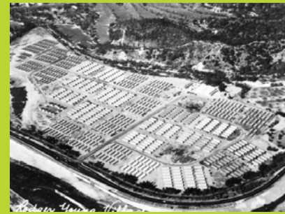
1946 Sweeping drafts and industrialization during WWII again lessen the prevalence of encampments. Upon their return, the Los Angeles City Housing Authority erected temporary huts in Griffith Park for veterans and their families. The area was razed and returned to park space in 1954.
