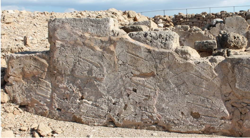
Figure 2.13: Herringbone incisions in the arriccio layer (base plaster layer) as preparation for subsequent plaster layers, from the House of Orpheus.
