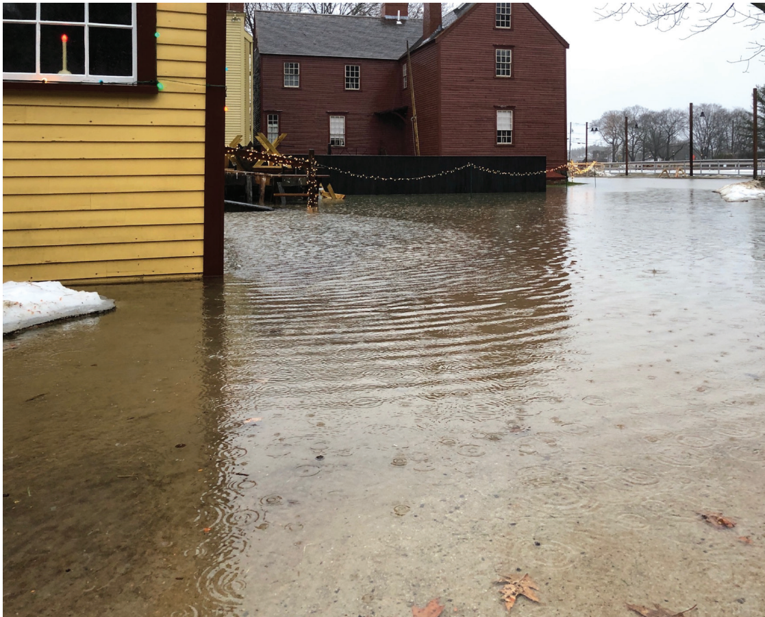
Infill flooding during high tide at the Strawberry Banke Museum in Portsmouth, New Hampshire. STRAWBERRY BANKE MUSEUM
