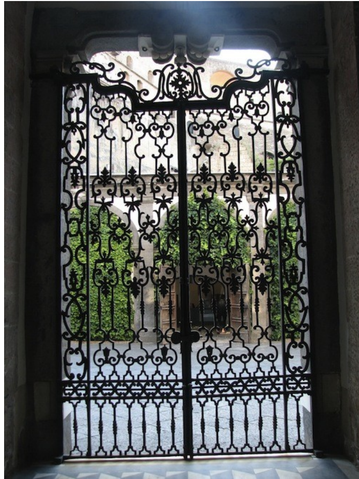
Fig 6 Naples, S. Martino. Entrance gate; probably of the late seventeenth century by Bartolomeo Antonio Picchiati or Luise Nauclerio. Photo © Helen Hills
