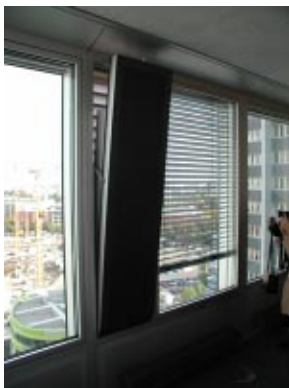
Exterior and interior view of the east triple-glazed facade system.
