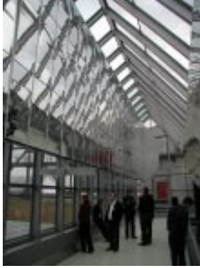
Light-redirecting skylight, Berlin.
