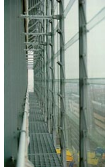
View from within the interstitial space.
