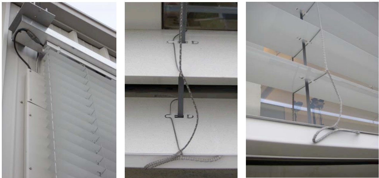
Figure 29: Views of header (below hoist beam), top of slat, and underside of slats.
