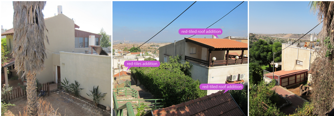
Figure 3.27 Houses in Alfei Menashe with pitch red tiled rooftops added on top of the original flat roofs. Photos by author.
