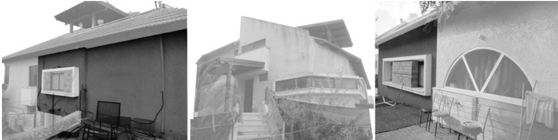
Figure 3.11 A renovated Ashcubit house in Beit Arye with two stories added—one on top and the other below the original Ashcubit house. Additions also include red-tiled rooftop, bay windows, rooftop balcony, arched window, and stone cladding. Remanents of the original, single-story Ashcubit house are painted in grey. Photos by the author.
