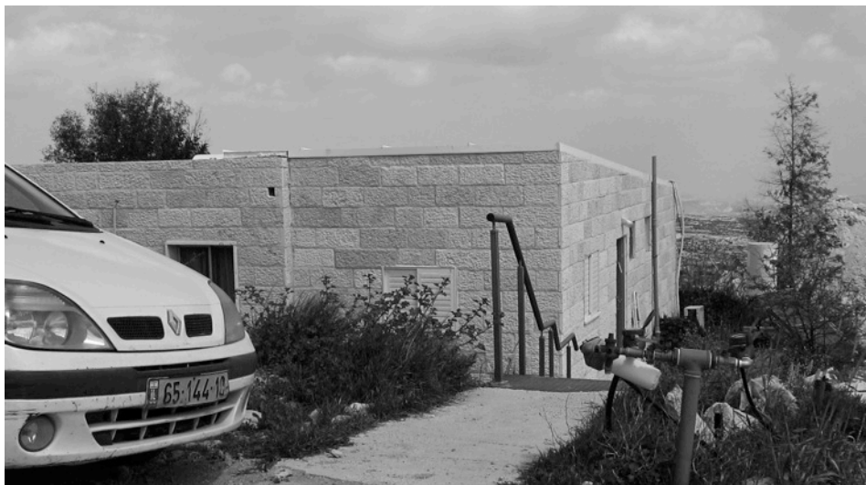
Figure 5.14 The portable placed on top of the covered concrete foundations. After some six months the couple started renovating the portable, they added rooms, a balcony space, and clad it with a thin layer of stone. Later, with time, they added more and more spaces, and today, in addition to their own unit, they have a rental one, all arranged around the original portable. Photo by the author.
