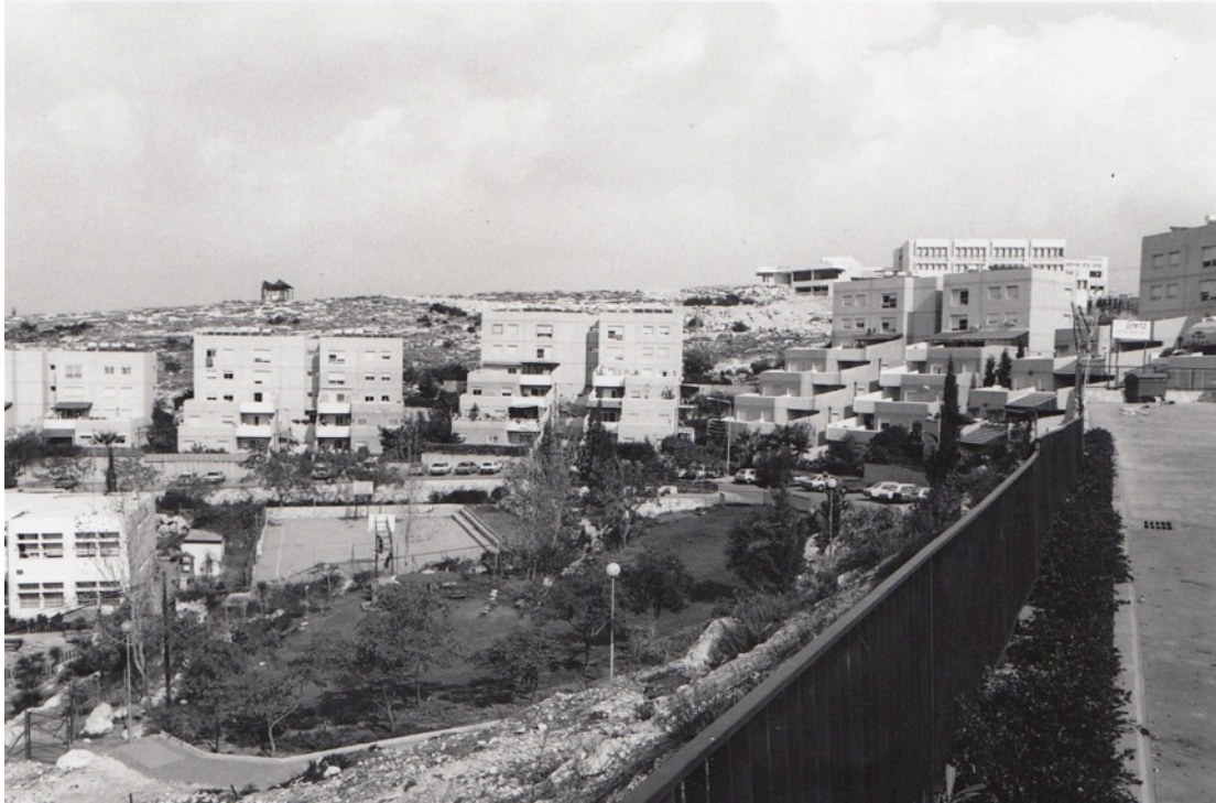
Figure 3.25 Low budget multistory buildings in Alfei Menashe, c.1986. Source: Alfei Menashe Archives.
