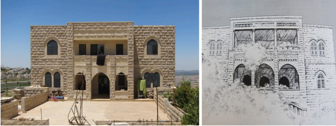
Figure 5.18 Shlomo's house in the outpost of Nativ Ha'avot (left) and an architectural drawing of Villa Harun al-Rashid, drafted by David Kroyanker, he consulted when replicating the building's façade (right). Other than some changes, such as moving the doubled windows from the second to the first floor, and lowering the ceiling of the upper balcony, Shlomo attempted to replicate the original façade with full earnest. Regardless of the obvious Arab origins of the house, though, he insisted it was a German Templers' house. Photo by the author.
