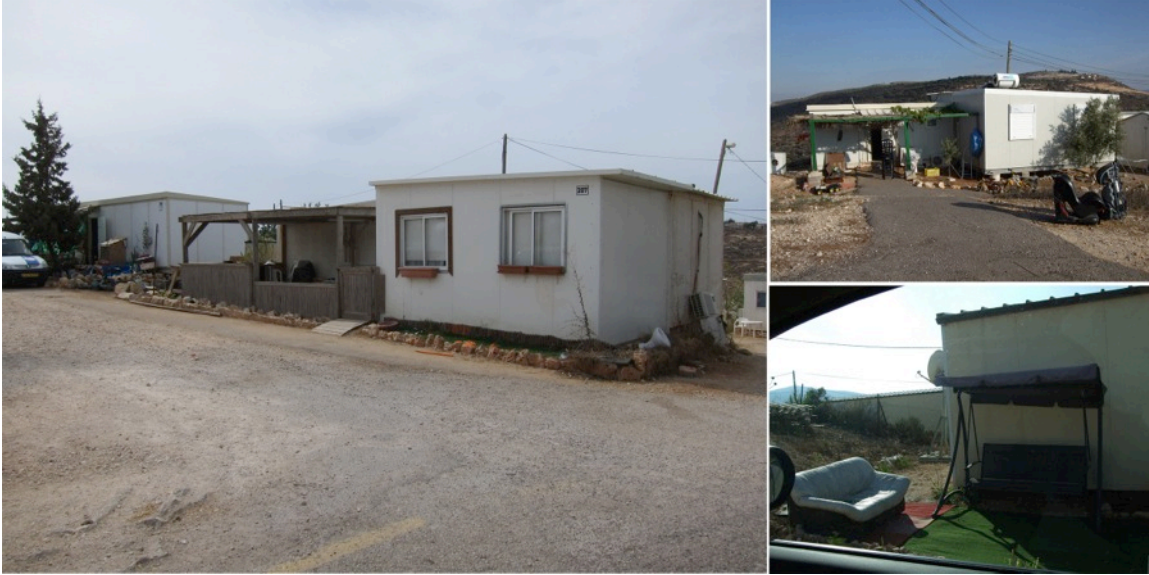
Figure 5.8 A portable with a roofed front porch in Pnei Kedem, 2015 (left). Portables in other West Bank outposts with different front yard installments, 2013 (right). Photos by the author.
