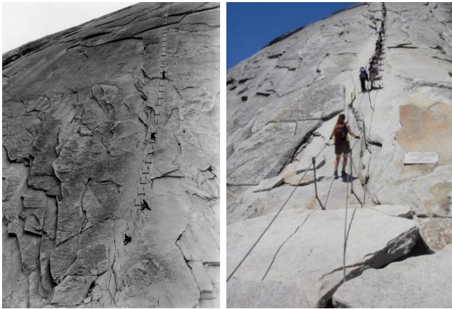
Image 1-2: Left: CCC workers replacing the cables on Half Dome, with new, heavier materials, 1932. Unknown photographer. Courtesy National Park Service, NPS History Collection, HFCA # HPC-000967. Right: the Half Dome cables in 2010, photograph by Jason Sampson.
