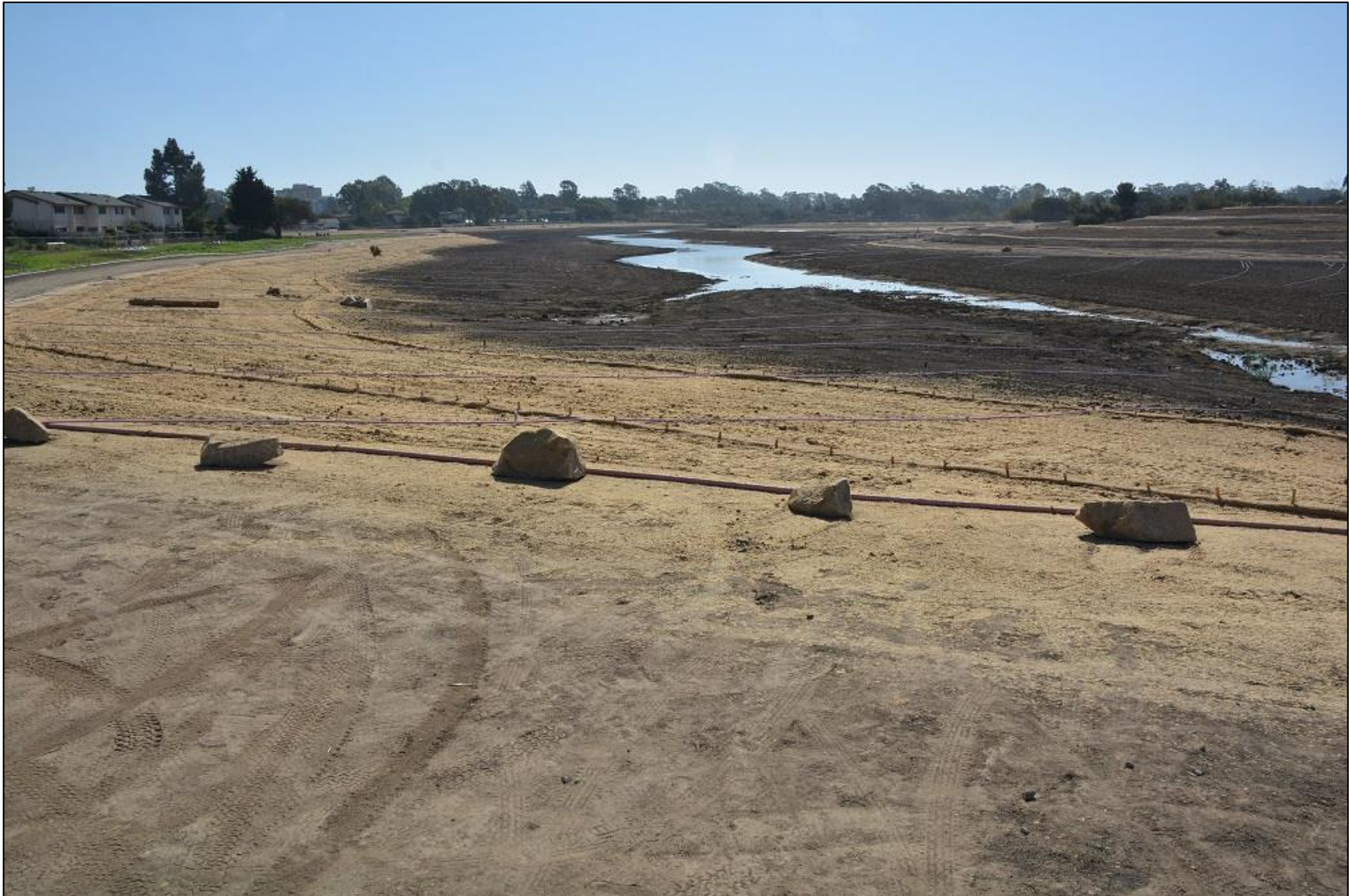
Baseline (post-grading) - October 2017
