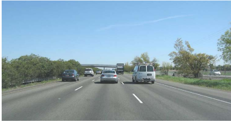
Figure 2.2. The test section on Highway I-80 east of Davis California with an OGAC pavement.
