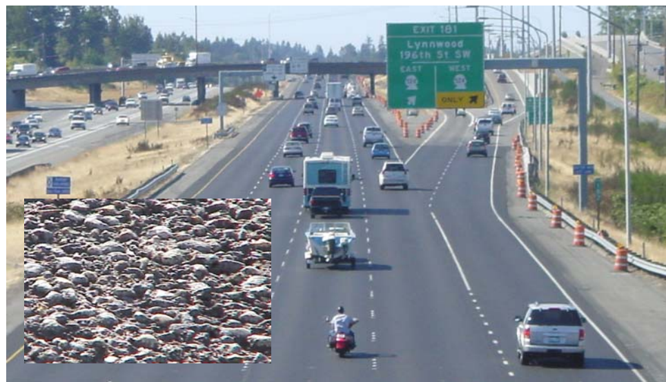
Figure 1.4. Interstate I-5 in Washington State where noise reducing pavements were constructed in June/July 2006 with a close up photo of a pavement after being exposed to studded tires (Photo Washington State Department of Transportation).
