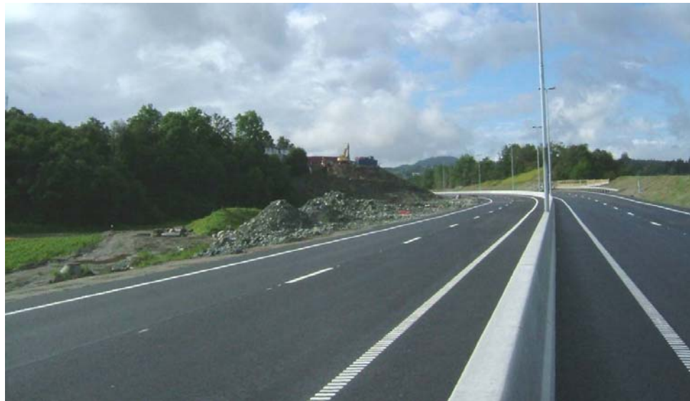
Figure 1.6. Road included in the CPX measurements carried out as a part of the Norwegian “Environmentally friendly pavements” (Photo Truls Berge, SINTEF ICT Acoustics, Norway).
