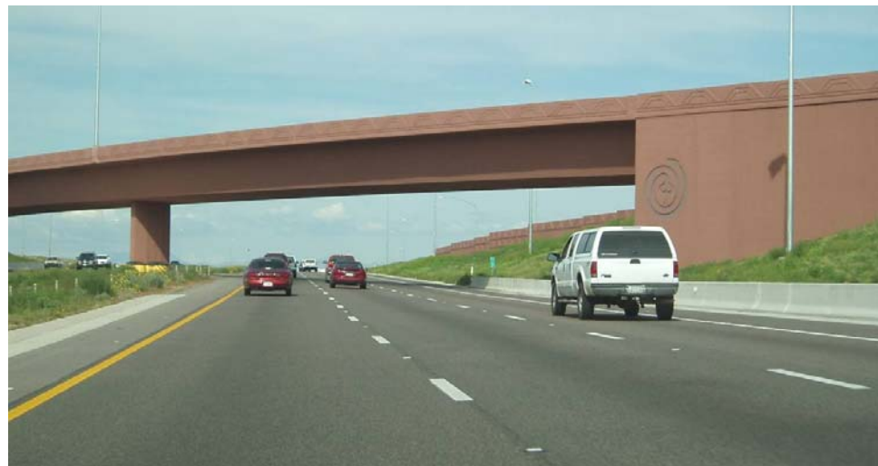
Figure 1.2. Asphalt-Rubber Friction Course (ARFC) has been used as a tool to reduce highway noise in Arizona.
