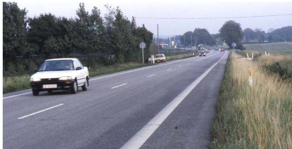
Figure 2.5. The test section at a highway near Viskinge in Denmark.
