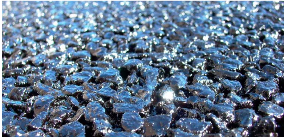
Figure 1.9. A one day old porous asphalt concrete (PAC) with a black bitumen film covering the aggregate prior to opening to traffic.
