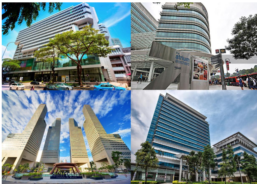
Figure 2. Four sample large office buildings surveyed in this study.
