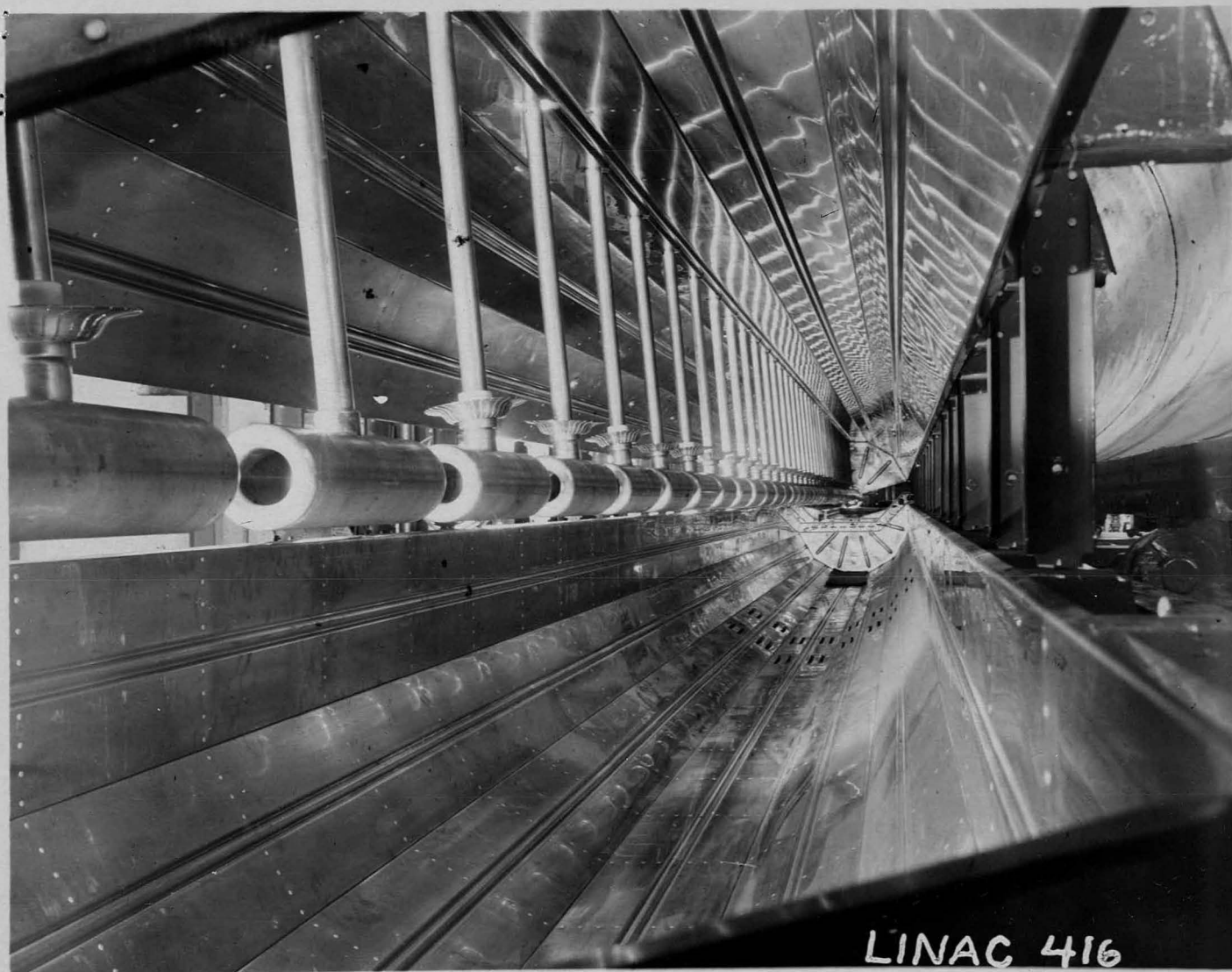
LINER OPENED UP AND STANDING ON EXTENSION LEGS TO PERMIT DRIFT TUBE ALIGNMENT
