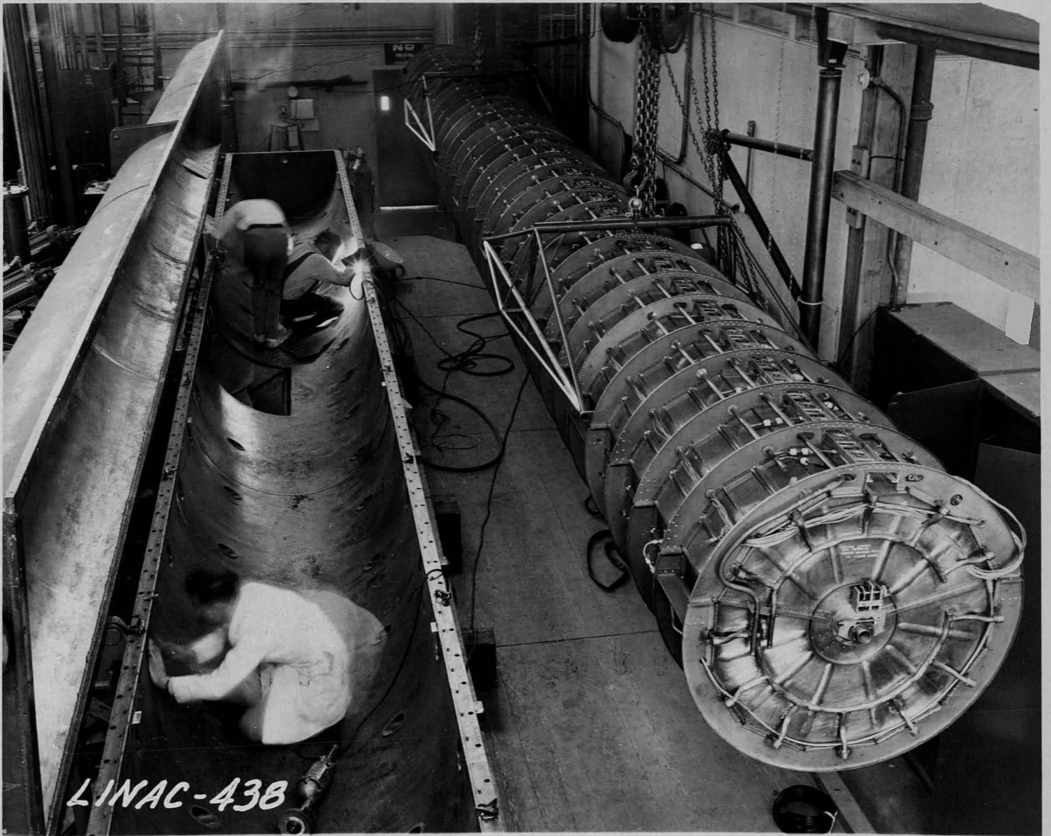
LINER SUPPORTED ON LIFTING FIXTURES FIG. 20
