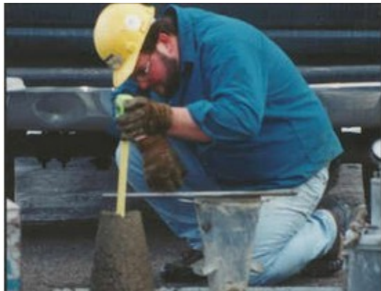
Figure 1: Slump test (Test concrete workability)
