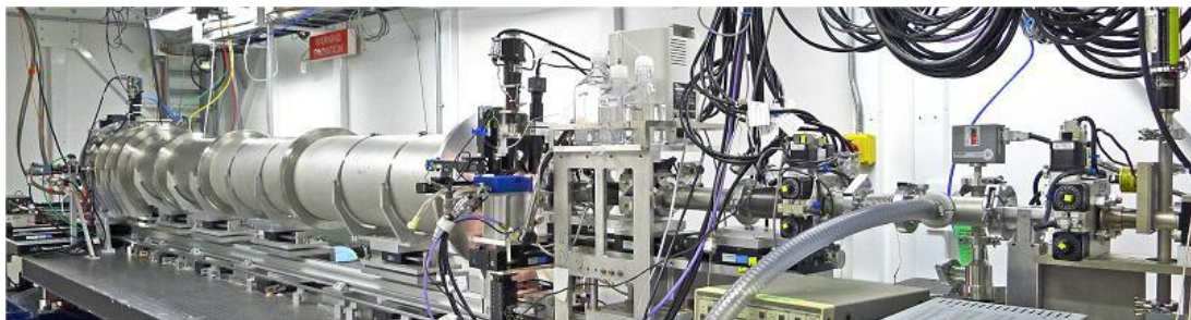
Figure 24: Beamline 4-2 hutch interior. The beam path follows the vacuum tube from the right through the sample chamber (not visible) to the area detector at the far left.
