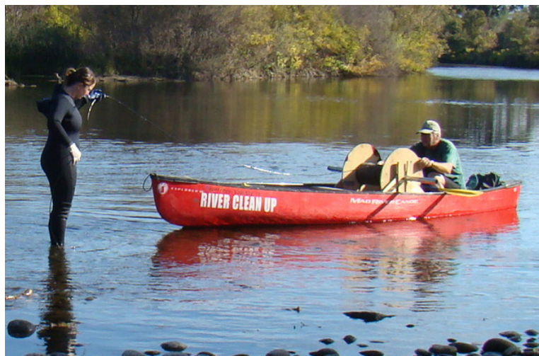
Erin Bray installs fiber-optic distributed temperature sensing cable (DTS) with the assistance of Chuck Kroeger (RiverTree Volunteers) along the length of a gravel bed reach of the San Joaquin River downstream of Friant Dam. Richard Sloan, RiverTree Volunteers
