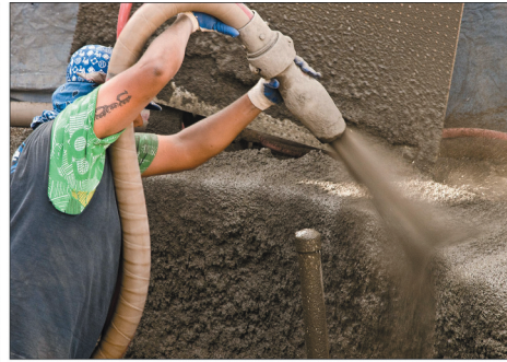
Contemporary Backyard Pool Construction with Gunite, 2011
