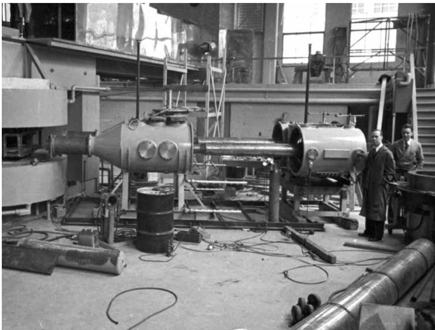
1939 > View of the 60" cyclotron used to generate the plutonium discovered in 1941. Members of the design team shown include (l) William Brobeck and Dale Corson. In 1937, at the age of 29, Brobeck became assistant director and chief engineer of the Lab. He oversaw the design and construction of the 60-inch and 184-inch cyclotrons, and finally the Bevatron.
