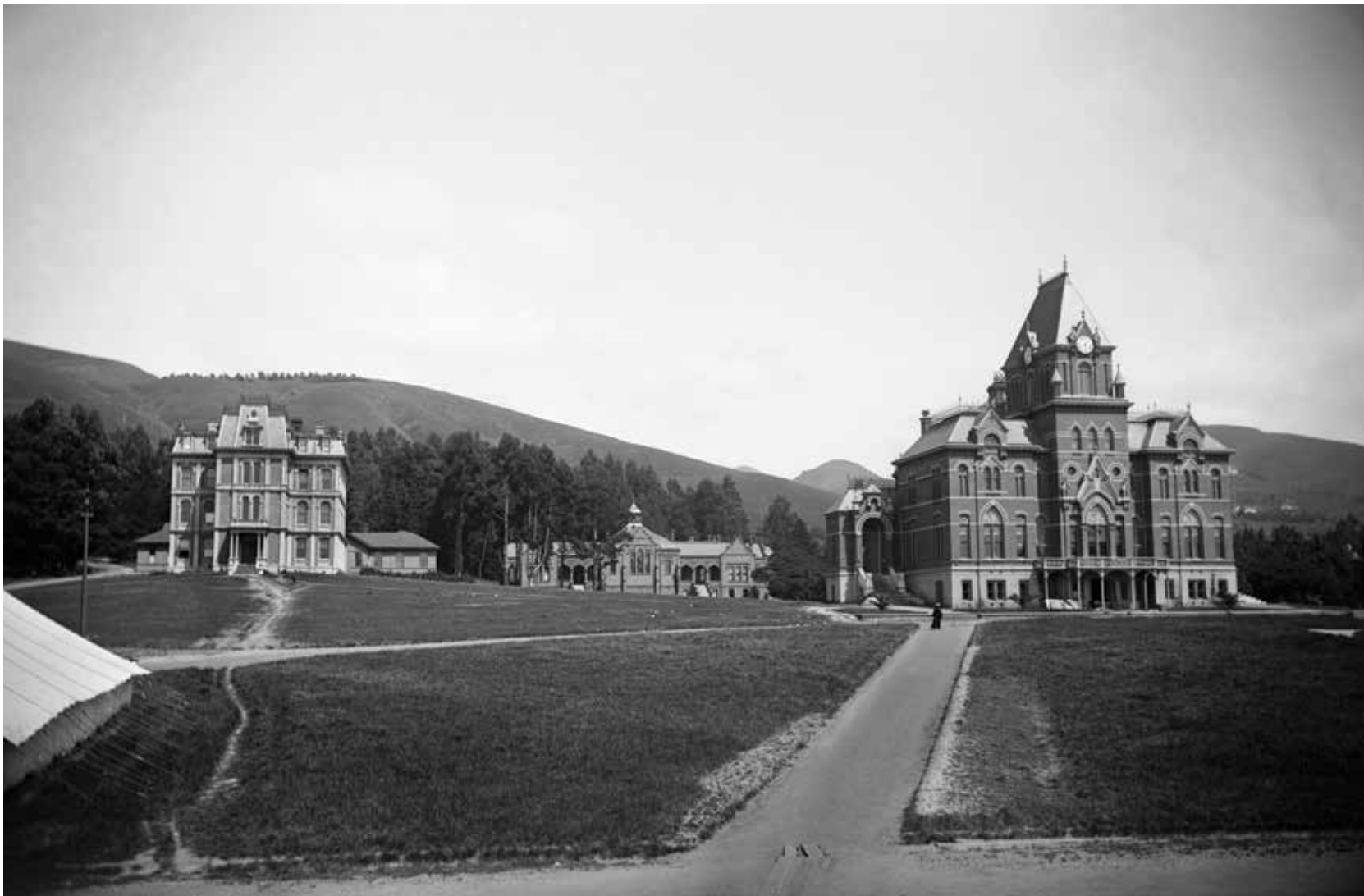
1897 > In 1891, a dedicated brick building (center) was constructed for the College on what is now the site of Hildebrand Hall and nestled between the first mining building (left) and Bacon Hall (right). It was designed by architect Clinton Day and constructed from 43,180 bricks. Additions were added in 1900, 1902, and 1912. Day designed some of San Francisco's finest buildings of the period, including the City of Paris building, Union Trust building, and Gump's department store.
