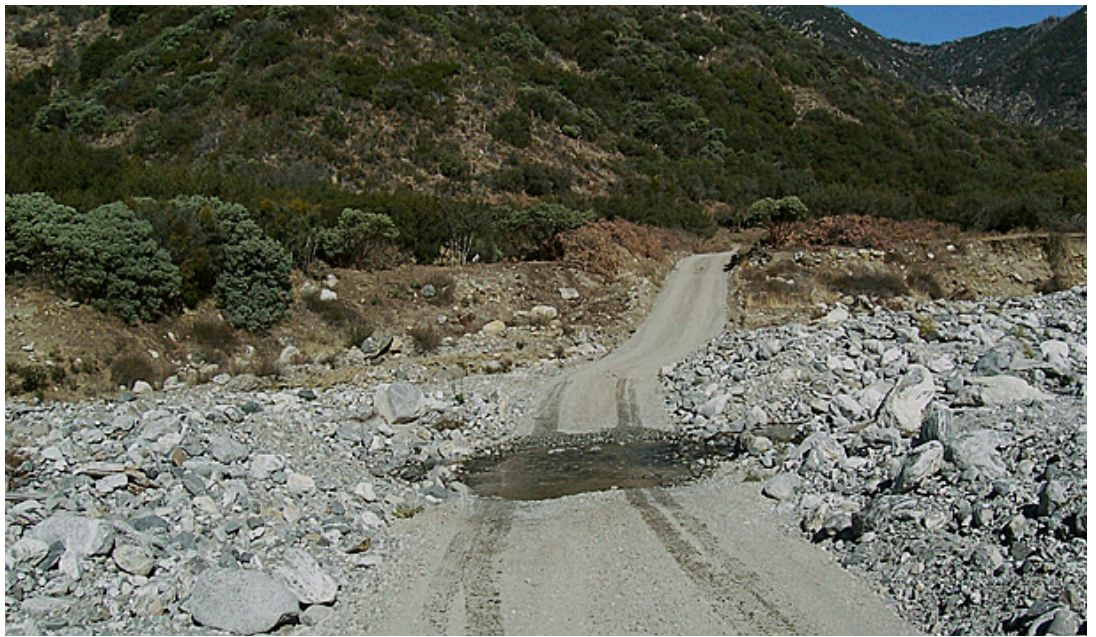
Figure 13. Wet ford stream crossing. These are sometimes called "Arizona crossings." Photo: Richard Harris.
