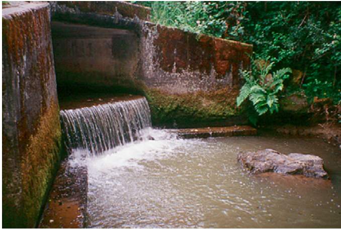
Figure 15. This box culvert will not permit fish passage because it is too high above the stream (excessive jump height for migrating fish) and the outlet velocity is too high (exceeds swimming ability of migrating fish). Any new culvert on a stream that supports fish must allow passage; many deficient culverts are being replaced. Photo: Richard Harris.
