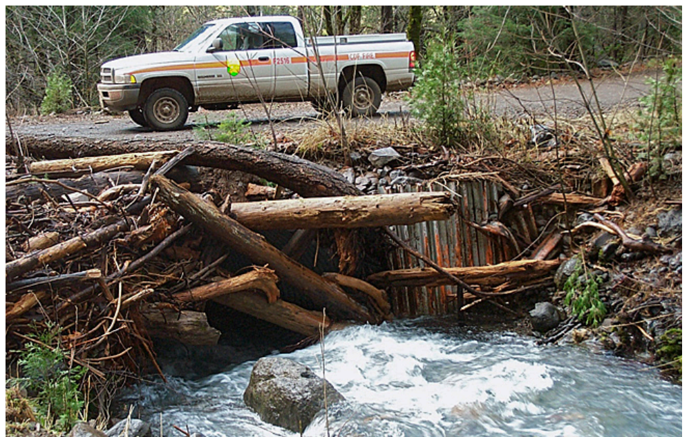
Figure 20. This extreme case of culvert blockage at a stream crossing was caused by a large storm event. All culverts should be inspected before and after storms to ensure that they are clear. Photo: © Angela Wilson; used with permission.
