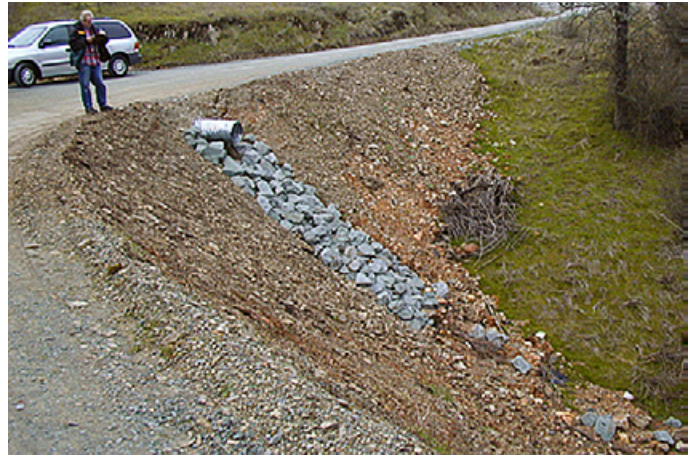
Figure 16. Rock has been installed at the outlet of this newly installed cross drain to prevent slope erosion or gullying. Photo: Richard Harris.
