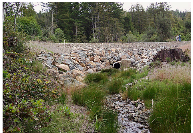
Figure 19. This reconstructed stream crossing on an all-season road used for hauling timber illustrates many desired design features. The culvert is sized to accommodate 100-year storm flows plus debris and sediment. It is located at the base of the road fill at the elevation of the channel to prevent scour. The face of the crossing fill is armored with rock. The road has a critical dip to prevent diversion and is surfaced with gravel.
