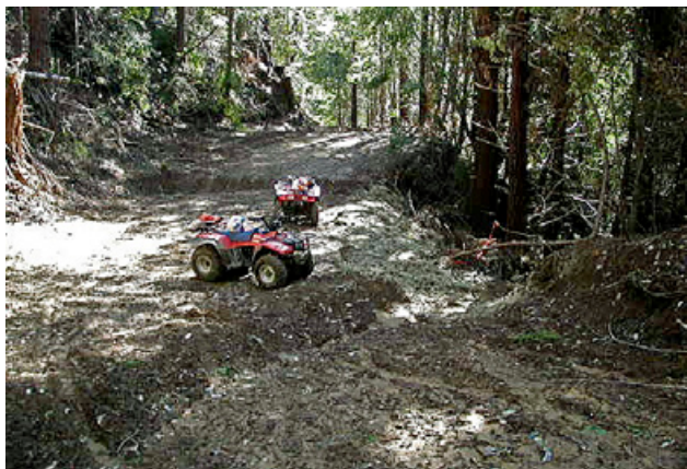
Figure 12. Water bars and straw mulch have been installed on this seasonal road prior to the onset of the rainy season. Water bars drain road surface runoff to prevent erosion. They will be removed when the road is put back in use. Photo: © Angela Wilson; used with permission.
