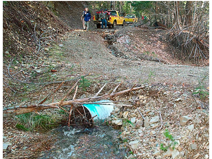
Figure 2. In this case, a culvert located uphill from the one shown plugged and diverted stream flow and sediment down the road into the stream. Photo: © Angela Wilson; used with permission.
