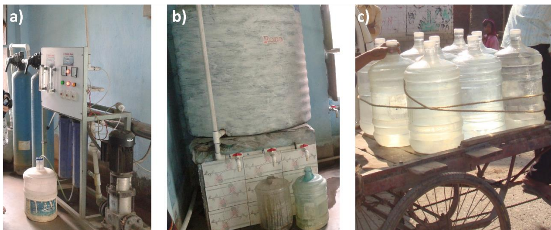
Figure 5-2: Production and distribution of 20 L containers of treated water in Area 1. a) Treatment unit including several filters and a reverse osmosis membrane. b) Storage tank and filling station. c) Distribution of treated water to households.
