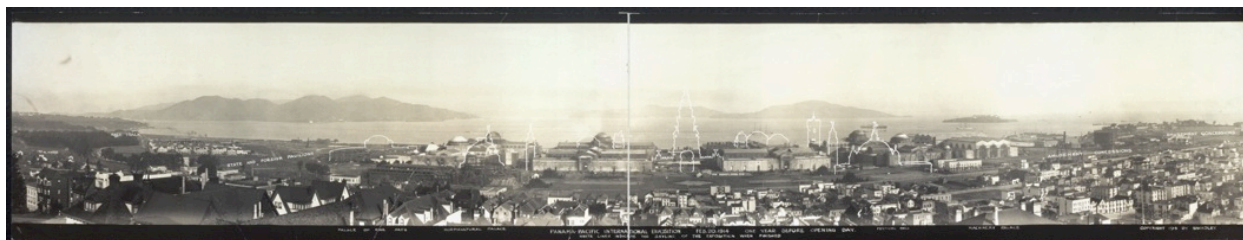
Figure 28. Panoramic photograph with silhouettes of anticipated fair structures, displaying the linearity of planning involved. Library of Congress, 1914.
