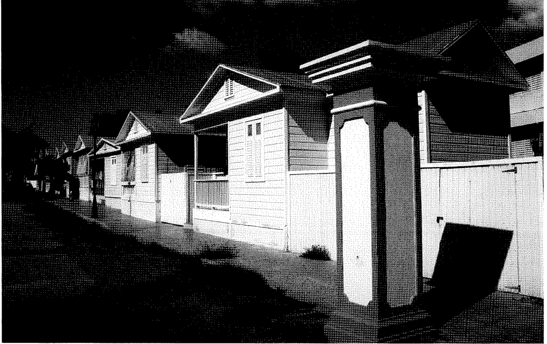
Restored working class casitas in Ponce, Puerto Rico.
