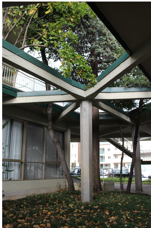
Fig. 13. Social services building, view from beneath the porch. Photo: Anastasiya Collins (2014).
