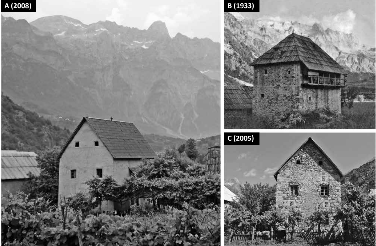
Figure 7.16. House in Theth-Ndrearj (ST245): (a) 2008 and (b) 1933. (c) ST245 as it appeared in 2005. Note window transitions over time and the continuing process of maintenance. Wayne E. Lee and Shan Pici, used by permission of the Fototeka Kombëtare Marubi, Shkodra, Albania
