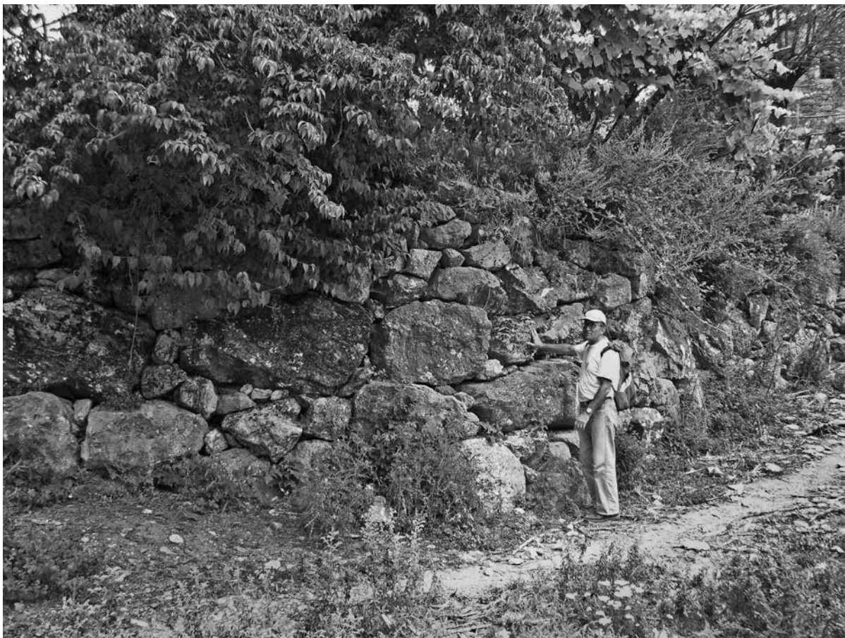
Figure 9.25. Large wall at EAS Site 010. Robert Schon
