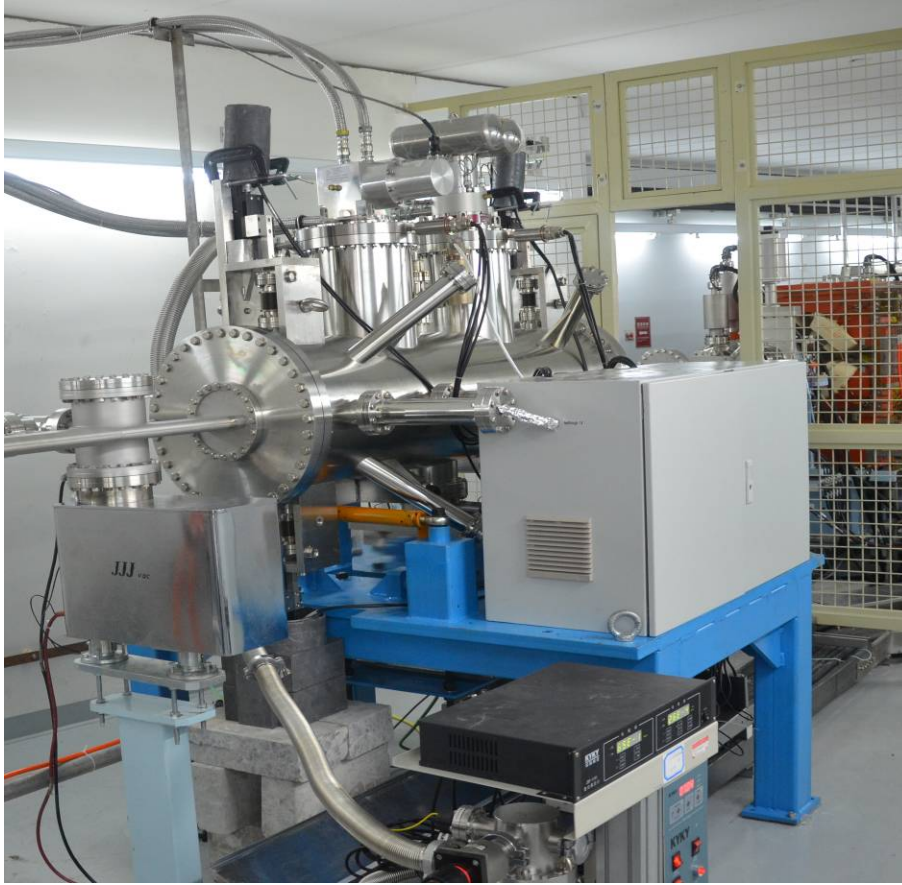
FIGURE 1 Installed calorimeter in storage ring
