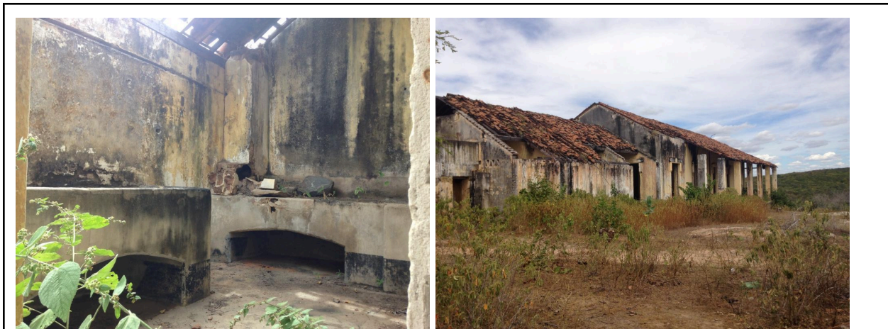
Figures 3.16 and 3.17: Current remains of the kitchen facility at the Patú camp, and the outside of the kitchen/main pavilion named as “the former Chief Engineer’s house,” where food distribution would take place.
