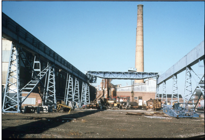
Figure 7. An outdoor crane bay in the shipyard of the Camden South Jersey Port of New Jersey. On the moving cross bar between the two rails, a block and tackle system can quickly place items anywhere in this storage yard.
