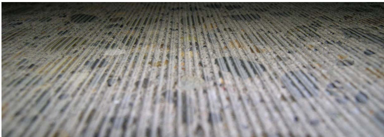
Figure 3.2: Concrete surface after the Next Generation Lite (NGL) grind.
