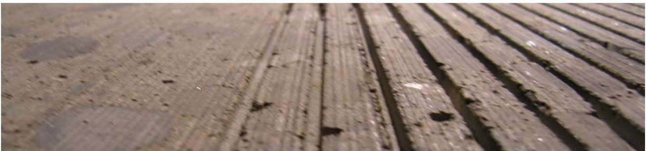
Figure 2.2: Concrete surface after flush grind only (left) and after grooving (right).
