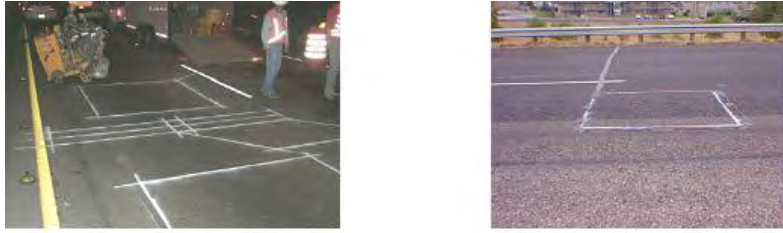
Figure 1.1: Installation of Inductive Loop Detector
