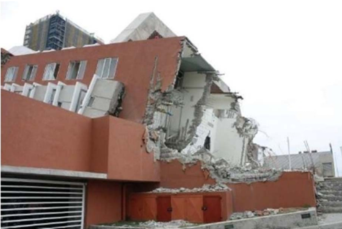
Figure 3.12 - Post-earthquake picture of Axis 5 (after IDIEM, 2010)
