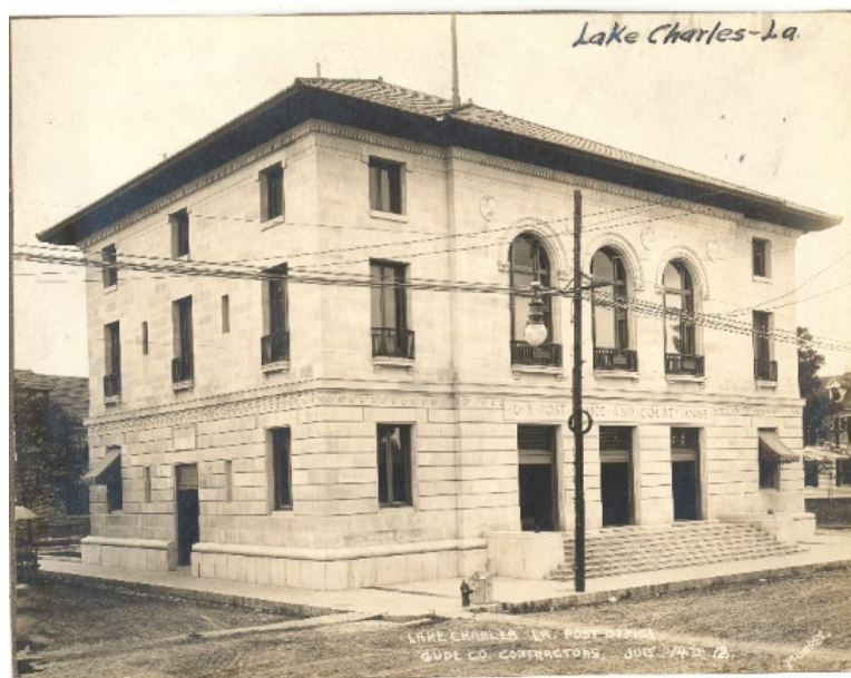
Figure 10: 1912 Lake Charles Courthouse
