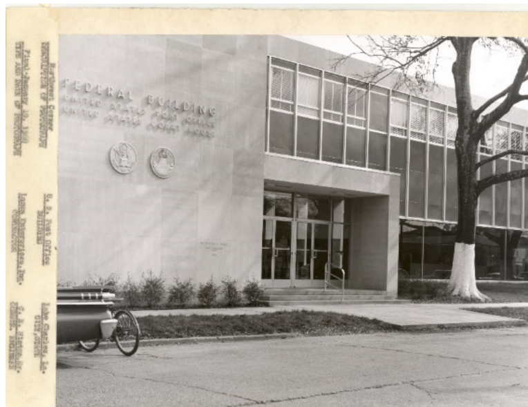
Figure 11: 1960 Lake Charles Courthouse
