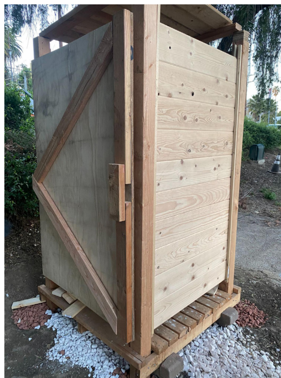
Figure 5-23. Hot water shower at Echo Park Lake. February 2021. Photo: Ashley Bennett.
