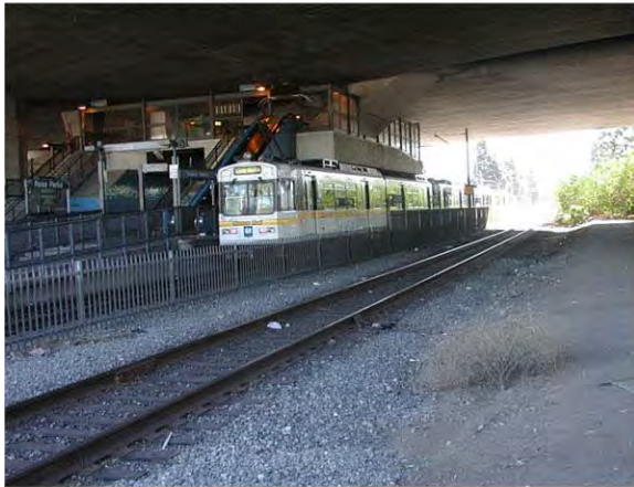
Blue Line Station Underneath I-105
