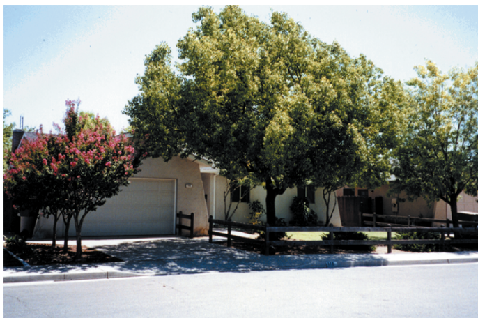
Figure 1. The test house, a single-story residence in Clovis, California, a suburb of Fresno.
