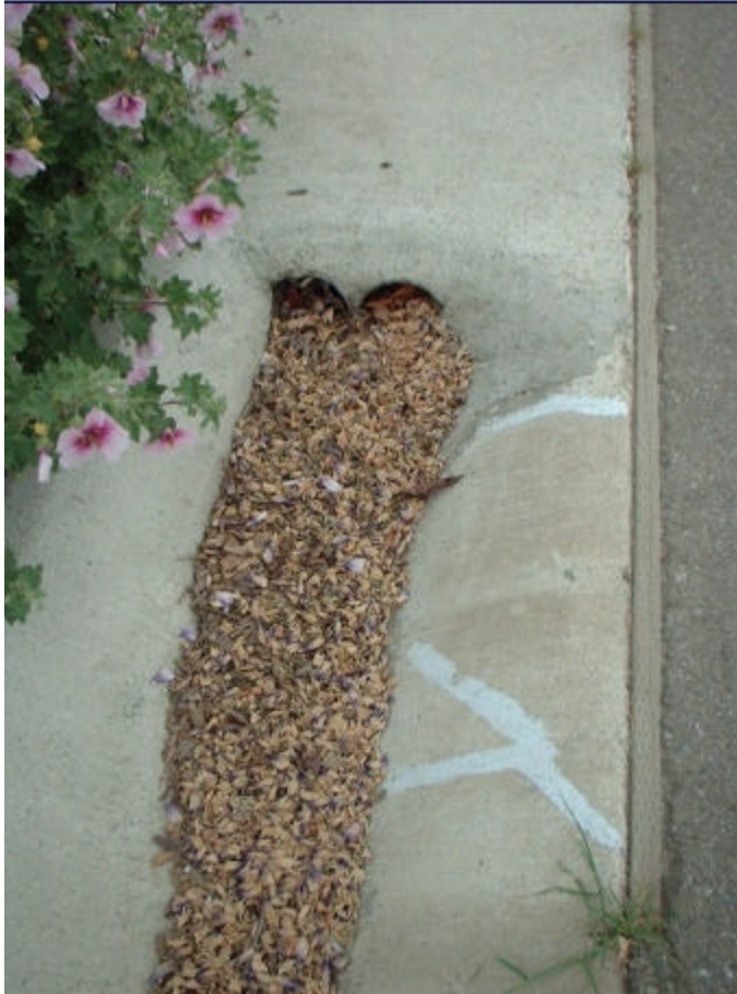
Figure 5: Pipes filled with debris at Tassajara Creek, 3/25/2004
