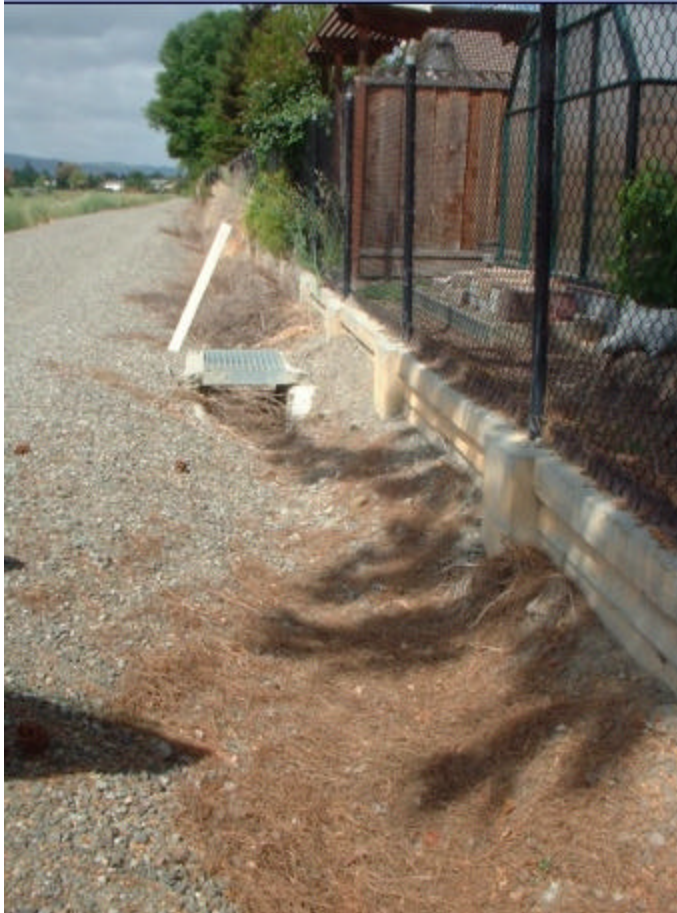
Figure 7: Earthen V-ditch at Arroyo Las Positas, looking downstream, 4/14/2004
